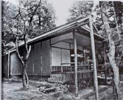
Contemplating this tree house at the Sells-Jaeger garden in Kyoto, Arthur came to a new understanding of the relationship between buildings and the natural world. (more... next page)
